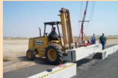
UF's low profile traffic barrier provides greater visibility, making roadways safer for drivers and construction workers
